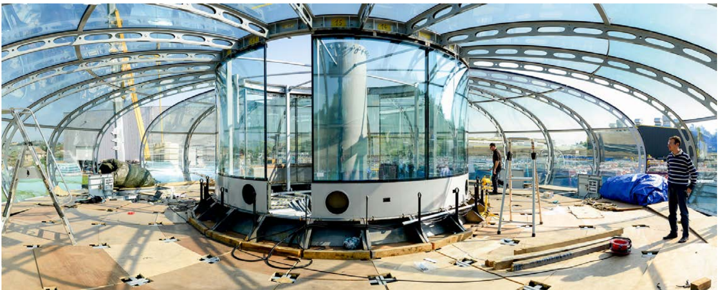
The i360 pod is attached to the two ring beams of this red chassis as it travels up and down the tower.
