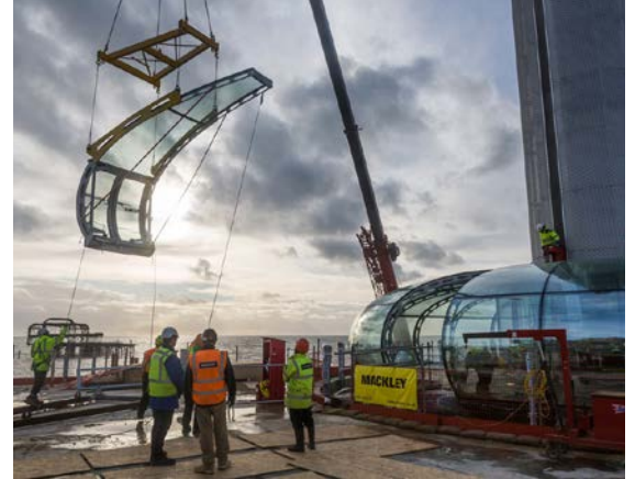
The last segment of the pod is lifted into place.
