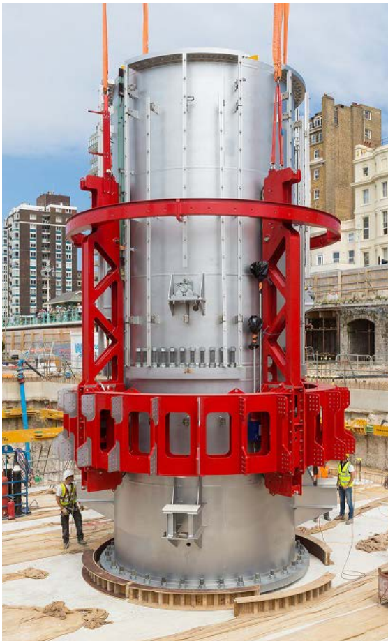
The i360 pod is attached to the two ring beams of this red chassis as it travels up and down the tower.
