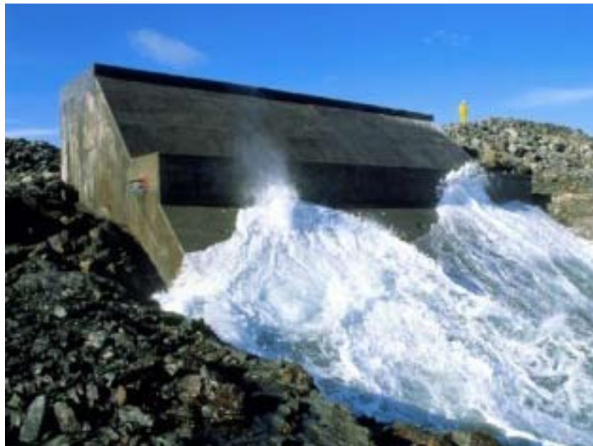
Another approach to wave power: this land-based wave power station generates enough electricity for 300 homes on the Scottish island of Islay.
