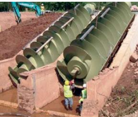
If a river has sufficient flow of water, two Archimedean screws can be installed side-by-side.
