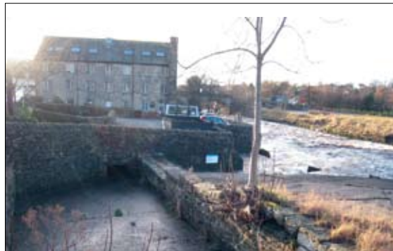
The mill race, the site chosen for Settle's micro-hydro scheme.
