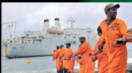
Bringing a SEACOM link cable ashore from the cable-laying ship.
