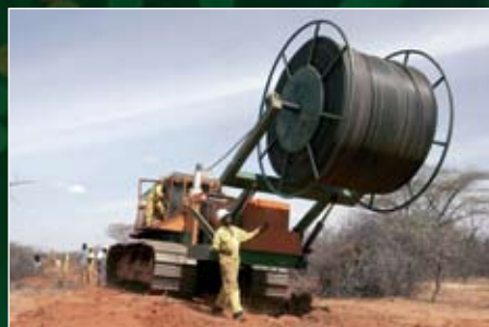
Laying the cable across rural Uganda.
