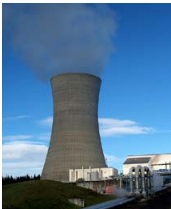
Rotorua geothermal power station in New Zealand
