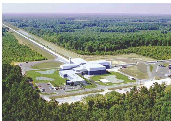
LIGO is the Laser Interferometer Gravitational Wave Observatory – here you can see the two long arms of the interferometer, at 90° to each other, used to detect ripples in space.
