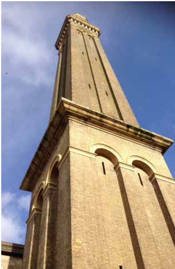
STANDPIPE TOWER AT LONDON MUSEUM OF WATER & STEAM
