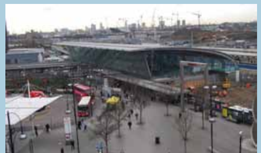
Stratford station, with the Olympic Park under construction beyond it.
