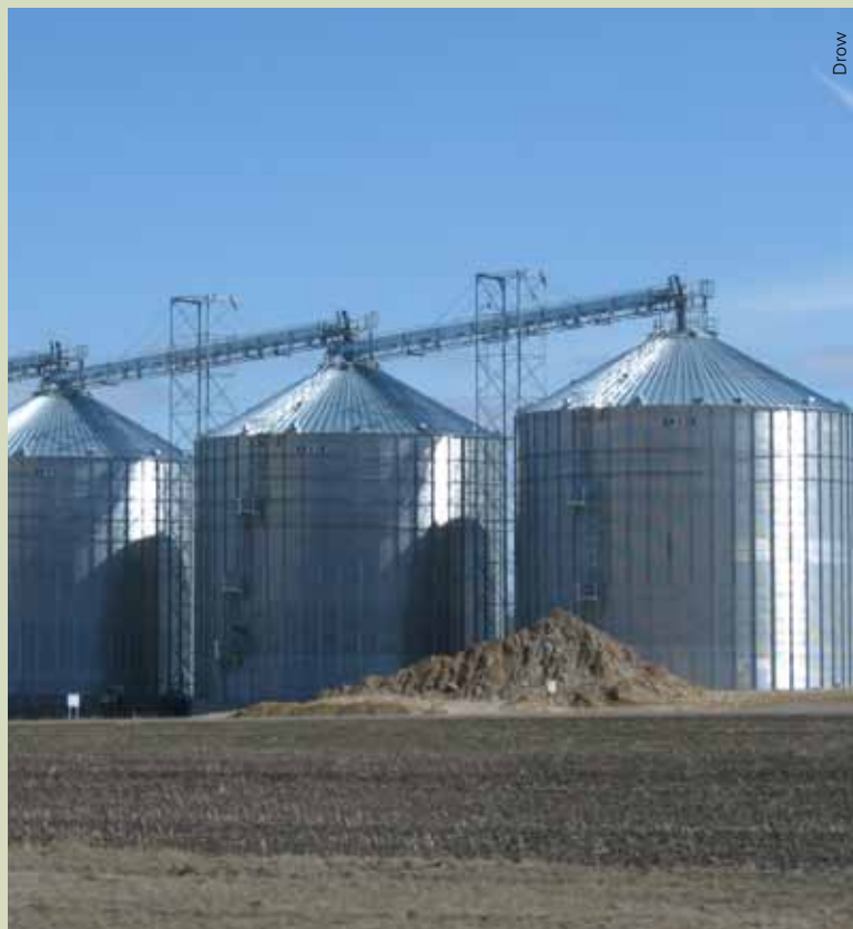
Silos in Wisconsin, USA, used for storing bulk quantities of cereal grains.
