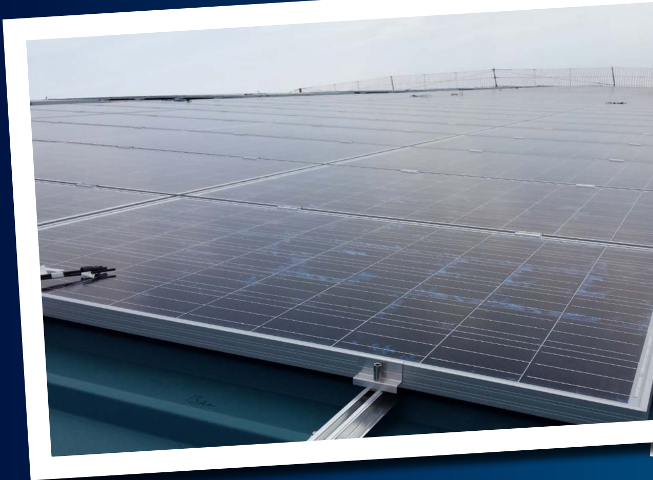
Panels cover most of the shed roof
