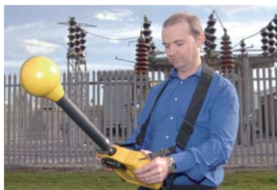
It isn't only nuclear radiation that needs monitoring. This detector measures the levels of electromagnetic fields near an electricity sub-station.
