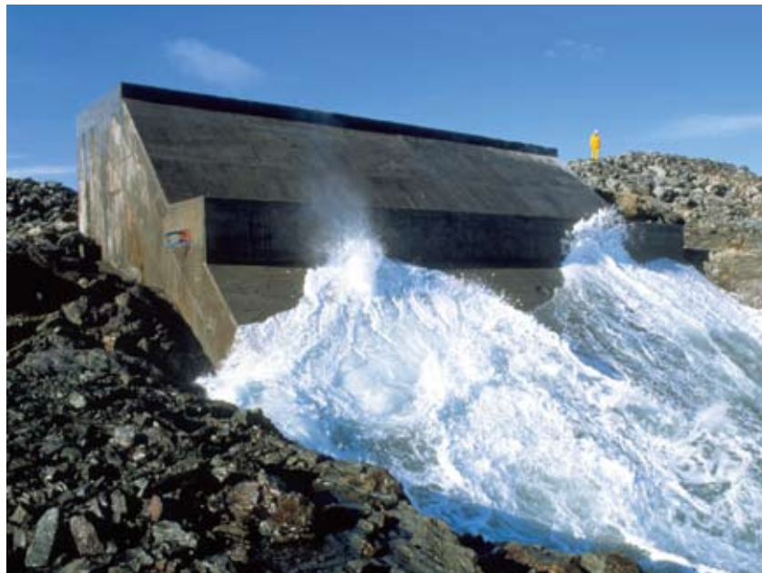
Another approach to wave power: this land-based wave power station generates enough electricity for 300 homes on the Scottish island of Islay.
