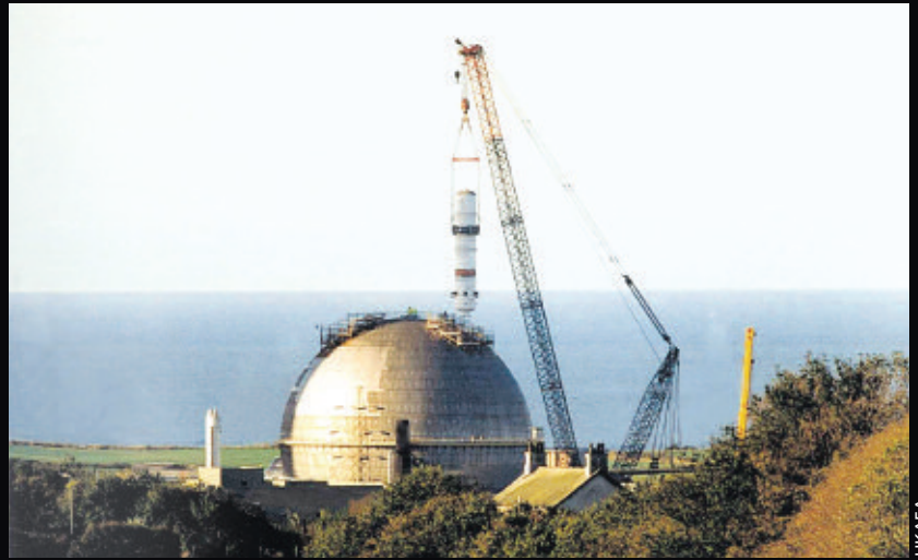
Removing the heat exchanger through the dome of Windscale's advanced gas cooled reactor using the world's largest crane. The metal could not be decontaminated so the entire exchanger has been buried in low-level waste disposal (an engineered trench lined with concrete)
